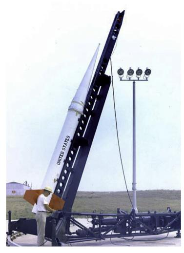
The Nike Smoke was a sounding rocket, part of a research project on the behavior of the horizontal winds in the upper atmosphere (about 75,000 ft), developed by NASA in the 1960s based on the Nike booster. The goal was to obtain more accurate data on the behavior of these winds in order to guide the design of new vehicles.
